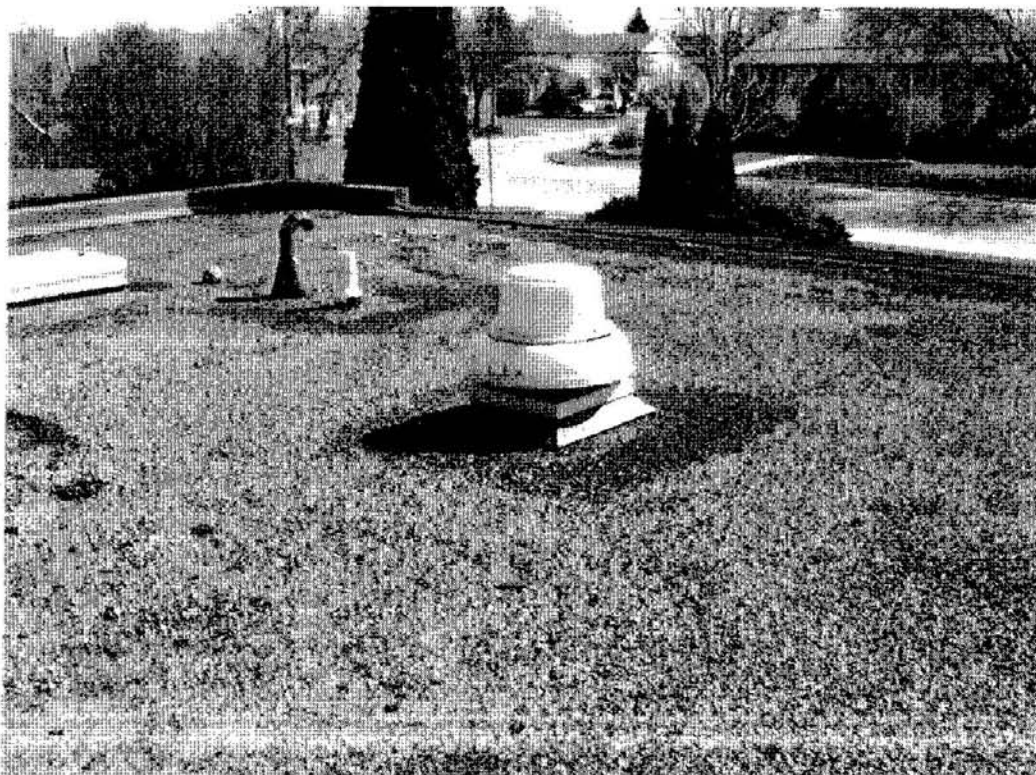
Photo 4. View of north east quadrant of roof.
